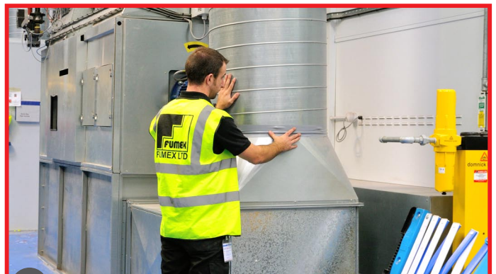
6 Inspect seals & ducting for leakage
